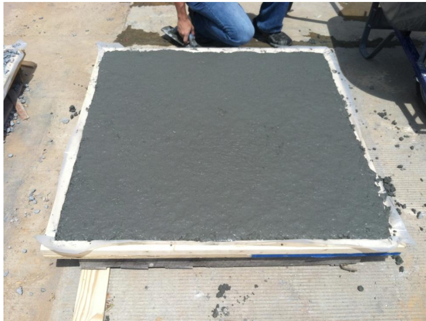
Figure 4.12 4' x 4' Test Slab
